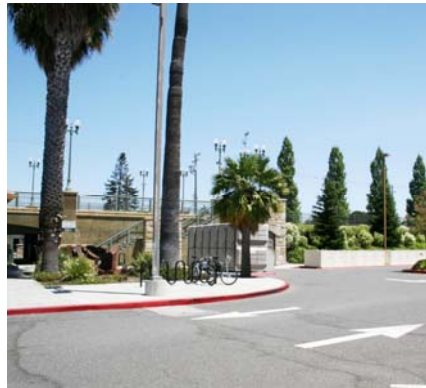
View of Bike storage and racks.
