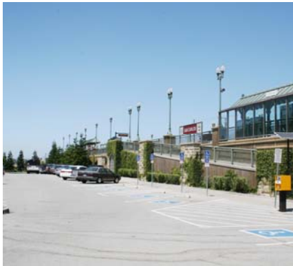
Caltrain station platform
